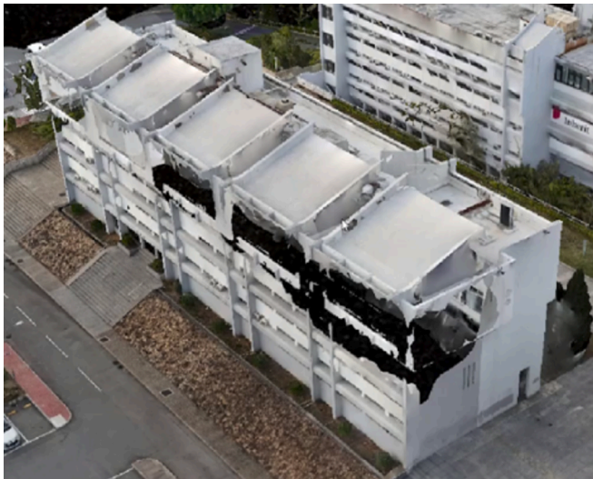
Fig. 3. Rough 3D point cloud model of the building.
